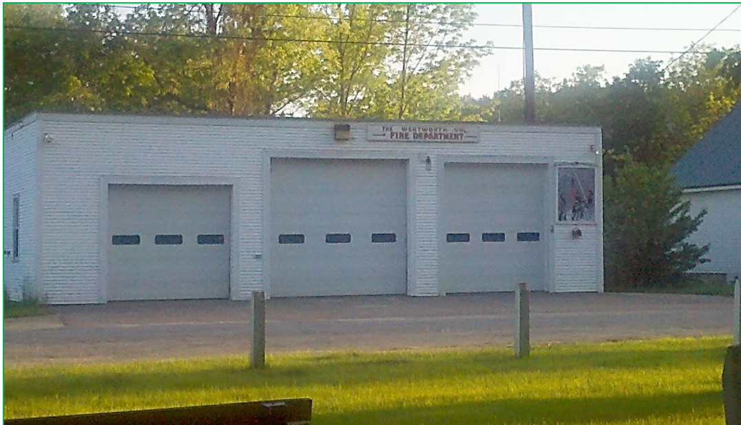
Wentworth Fire Station Photo Credit: MAPS
