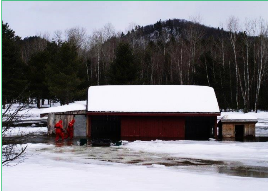
Wentworth Flooding, Tropical Storm Irene Photo Credit: Town of Wentworth
